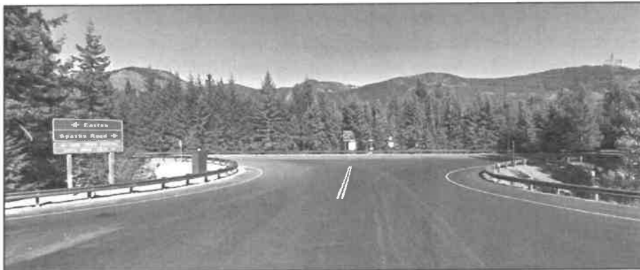
Figure 3: View Toward Site from I-90 Exit 70 Interchange
